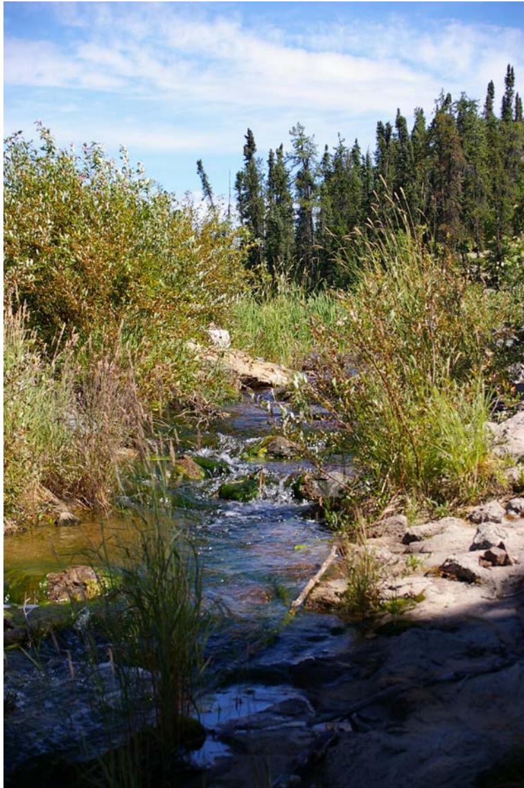
Photo 1 – Marie Reservoir Spillway looking upstream
