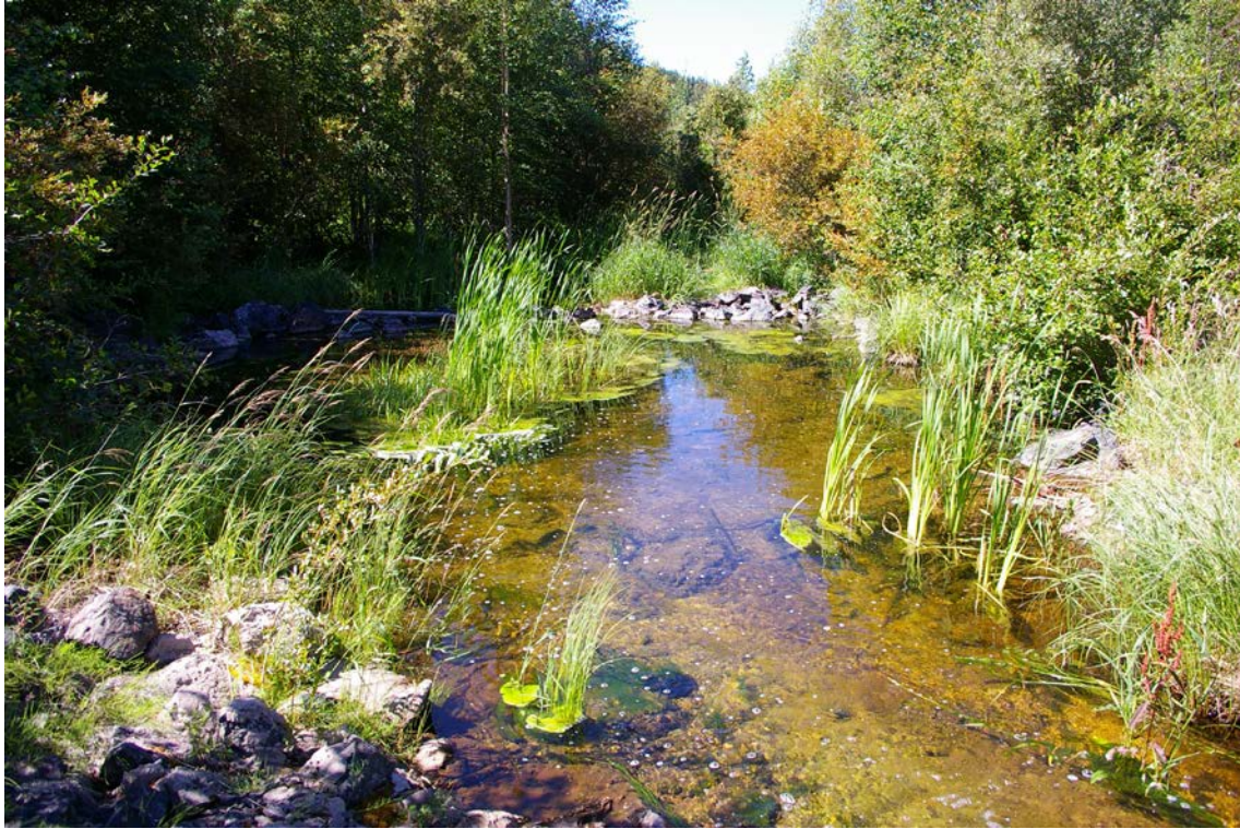
Photo 2 – Marie Reservoir Spillway (water flowing into stilling basin)
