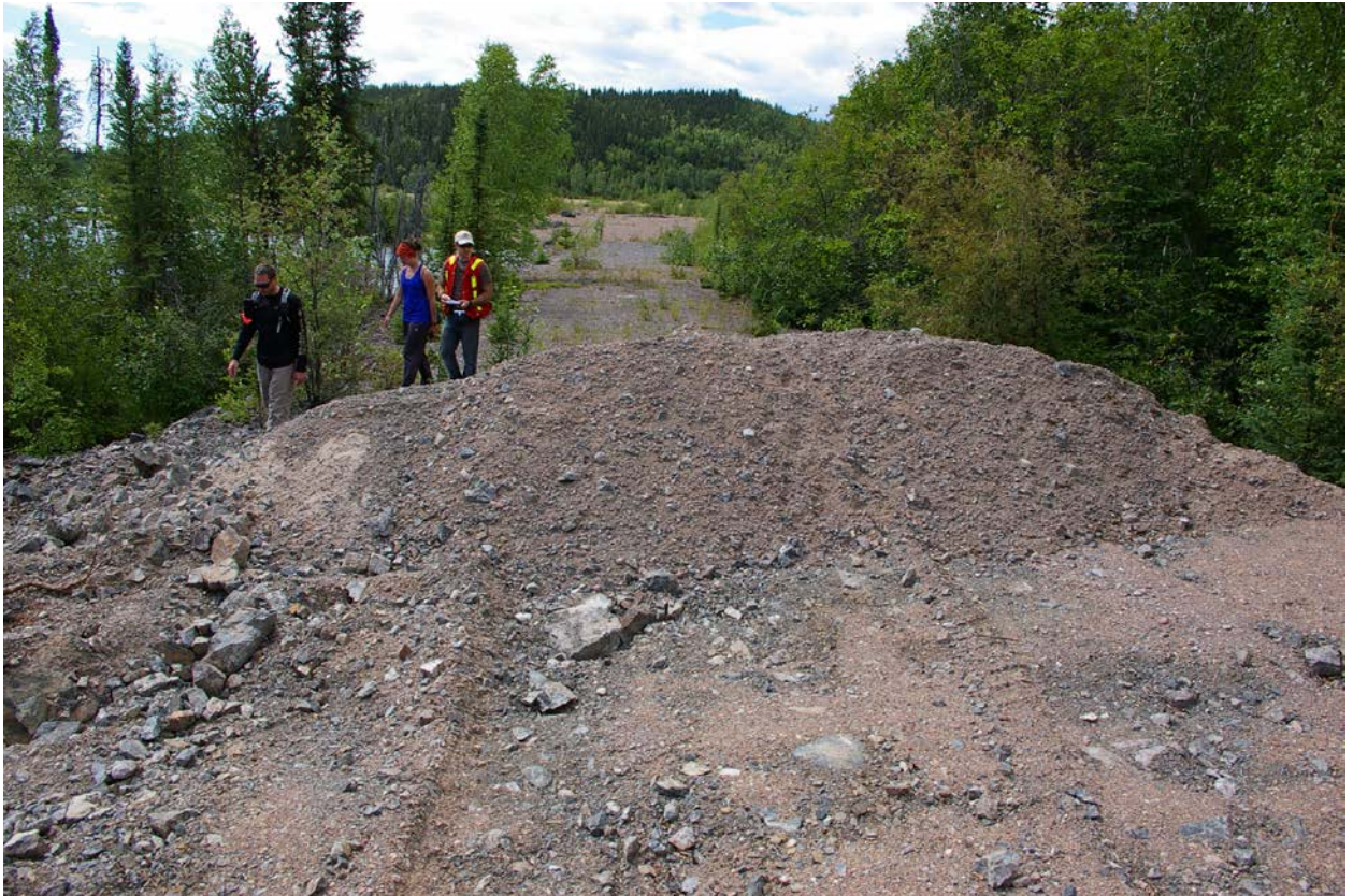
Photo 12 – East berm (looking west) repaired to prevent vehicular traffic
