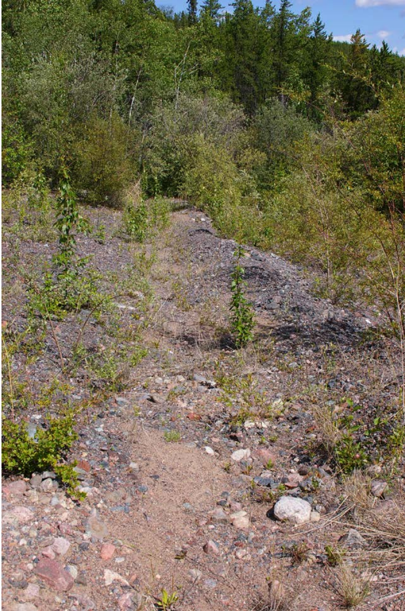
Photo 11 – Run-out structure along north access road
