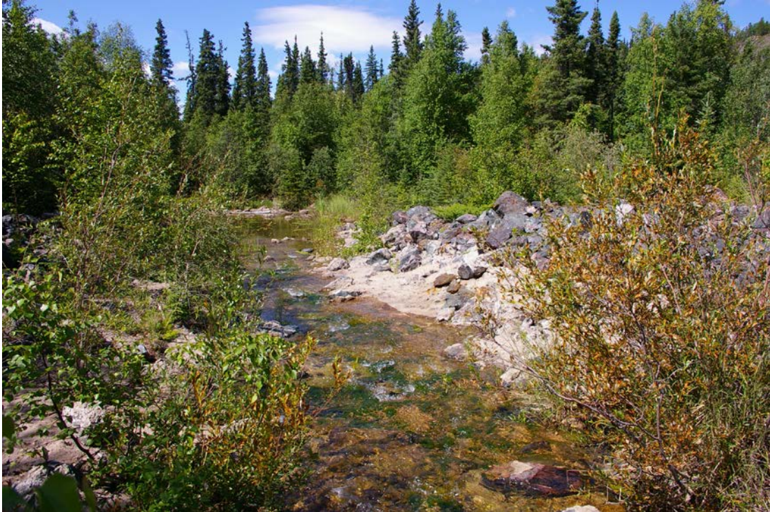
Photo 5 – Fookes Reservoir Spillway looking downstream towards the stilling basin
