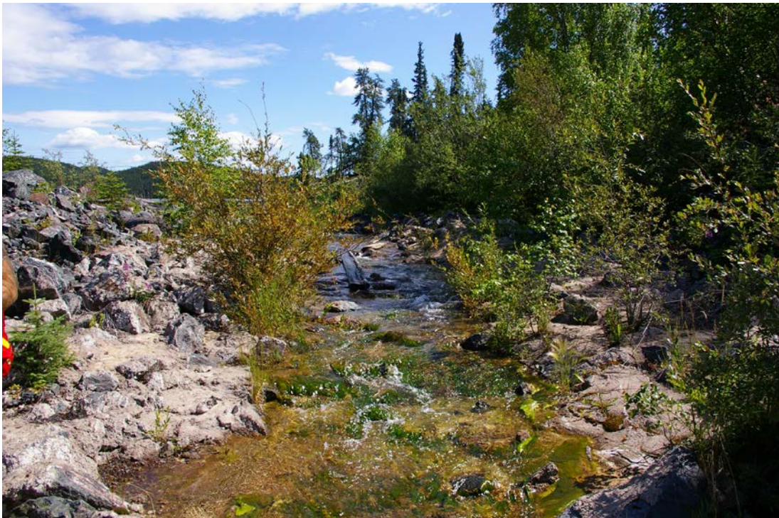
Photo 4 – Fookes Reservoir Spillway looking upstream
